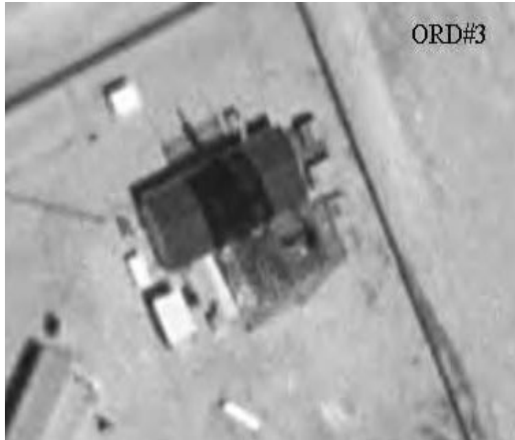
Figure 16. Aerial View of ASR-9, ORD #3, Oak Forest, Cook County, Ill.
